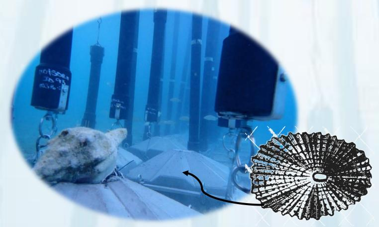
A **foundation design** based on nature, as the limpet, our foundation is designed with its radiused angularity; to resist tidal flow or wave action turning it over, we have adopted this for the concrete limpet shaped blocks which hold our barriers in position. Note the large sea snail taking up residency on this new barrier installation.
